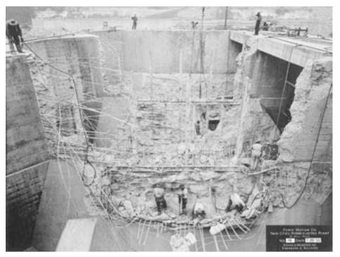
Ford had to substantially demolish the foundation for the hydroelectric plant built by the Army Corps of Engineers to allow for the installation of more advanced turbines, as seen in this photograph from July 1923. Photo courtesy of the author.
