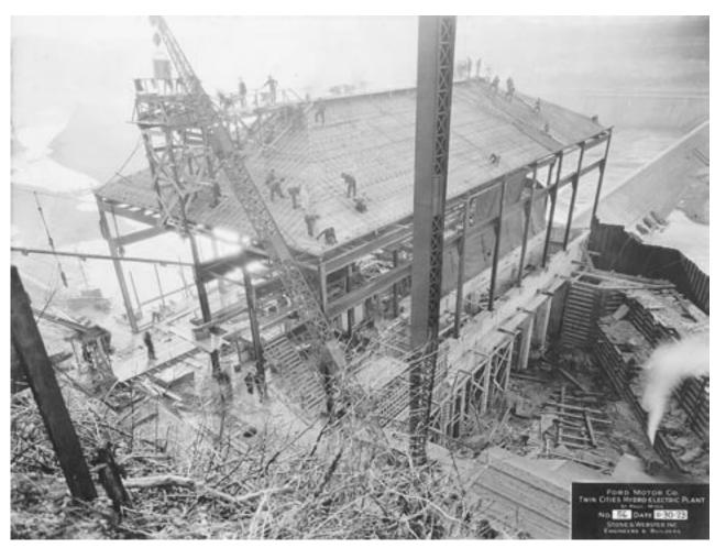
By November 1923, the structural framework for the new hydroelectric plant was installed. Photograph courtesy of the author.
